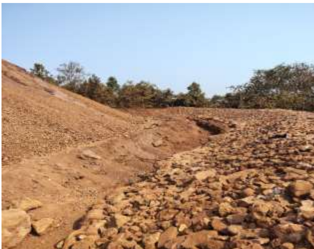
Photo-9 Garland drain at the toe of OB dump at Block II area
