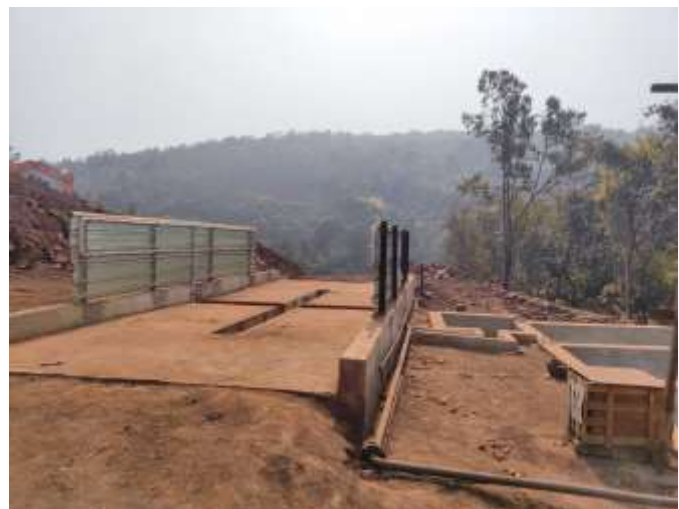
Photo-3 Wheel wash facility at the exit gate of Mines with recirculation system
