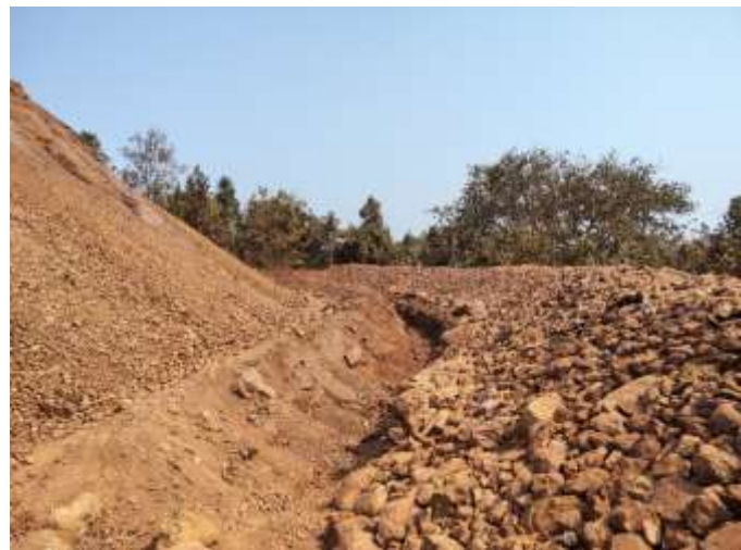
Photo-9 Garland drain at the toe of OB dump at Block II area
